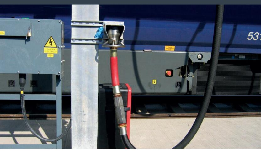
The IFC Flyte Coupling is used for the refuelling of trains in rail service depots. This dry disconnect type coupling has a 1/2" BSP threaded inlet and is designed to fit onto a standard 1-1/2" BSP threaded fuel hose.
